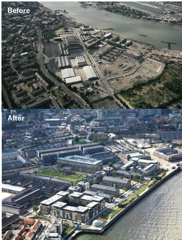
Figure 1: Royal Arsenal, before and after the regeneration © BHL
