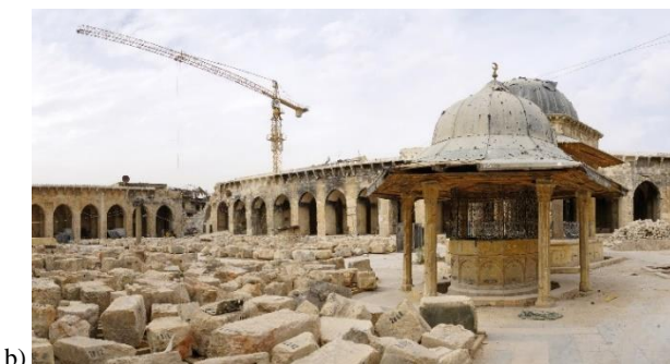
Figure 13. The Minaret of the Great Umayyad Mosque before the war and after the war. The blocks placed on the floor of the court, are numbered, raised with the visible crane and then photographed to proceed with the identification.
