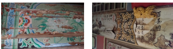
Figure 1. Painting was damaged by micro-climate change
