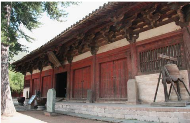
Fig.1 The East Main Hall of Foguang Temple
