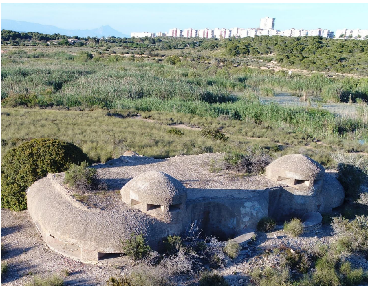
Figure 3. Current photograph of the main bunker (CG-BK04.elc) taken from the drone; in the foreground the southern front with various defensive elements (loopholes, hatches and pits); behind are the hills of Arenals and Cabeçó, the tourist developments and, in the background, the Puig-Campana in the mountain ranges north of the province of Alicante (photo: authors)
