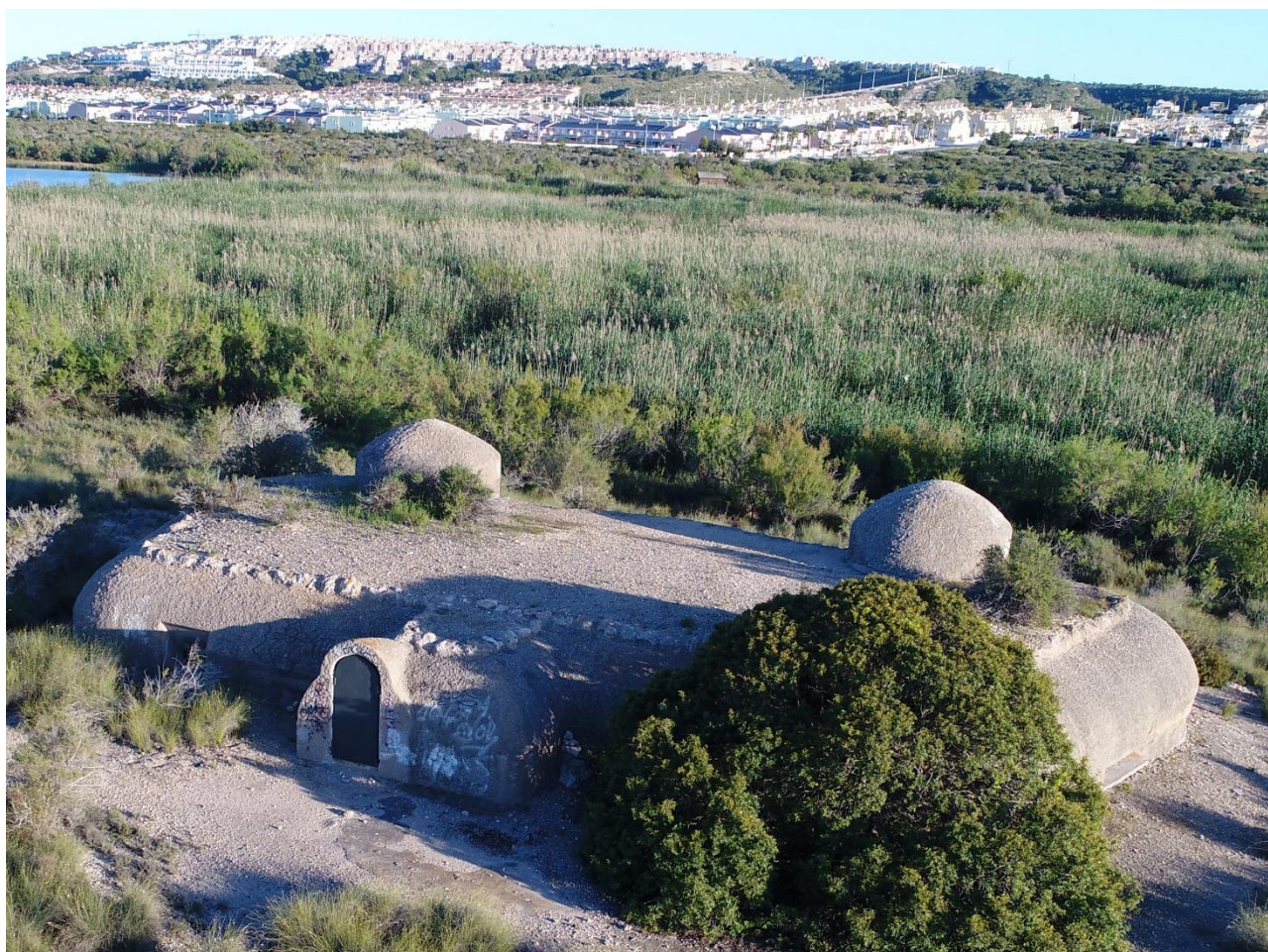
Figure 4. Current photograph of the main bunker (CG-BK04.elc) taken from the drone; in the foreground the northern front of the bunker with the only access to its interior and the upper surface (with the volumes of the hatches protruding); behind, the lagoon and, in the background, the tourist urbanizations on the mountain range and the cape of Santa Pola (photo: authors)
