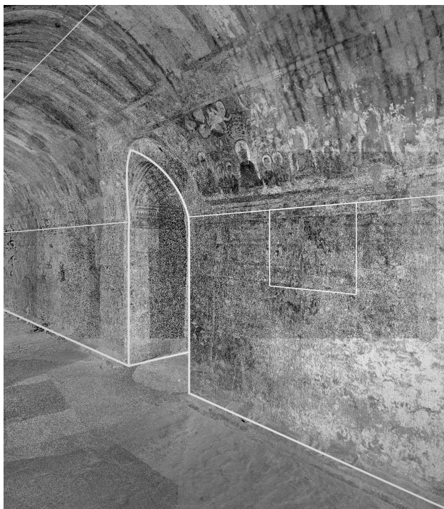
Figure 11. Laser scan in BIM of west wall painting.
