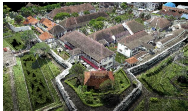
Figure 12. Integration of TLS and UAV pointclouds data by using Iterative Closest Point (ICP) algorithms
