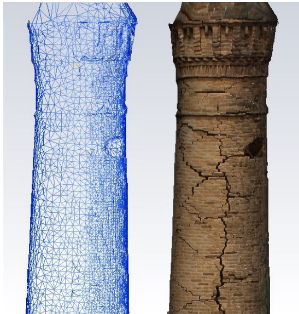
Figure 5: Detail of the TIN model and texturing (source: prepared by the authors)
