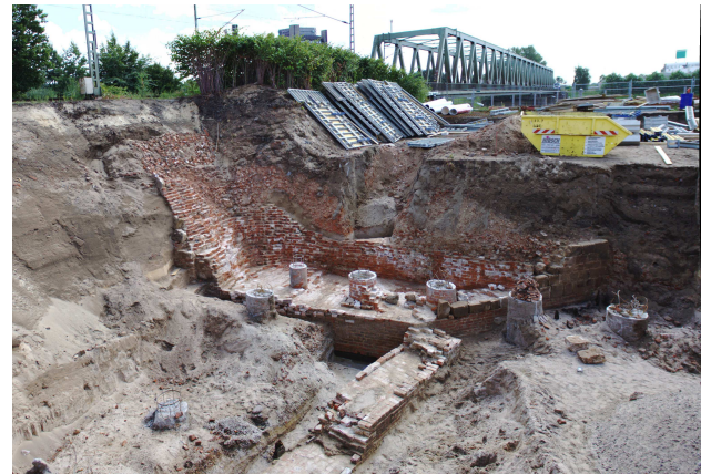
Figure 5. Excavation of the rediscovered Stephanitorzwinger in Bremen, Germany.
