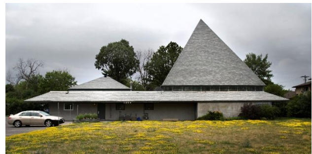
Figure 8. Ottawa East SDA south facade
