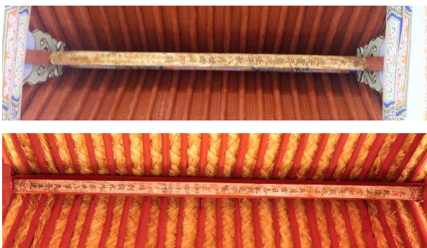
Figure.10 inscribed verbal contents under the ridge purlin in Wenchang pavilion and Stage building
