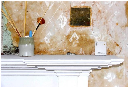
Figure 6: Conservator revealing the painting underneath the wallpaper above the fireplace. Source: Ann Shaftel
