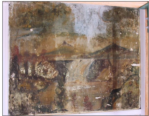
Figure 9: South wall layers of paintings. Source: Ann Shaftel
