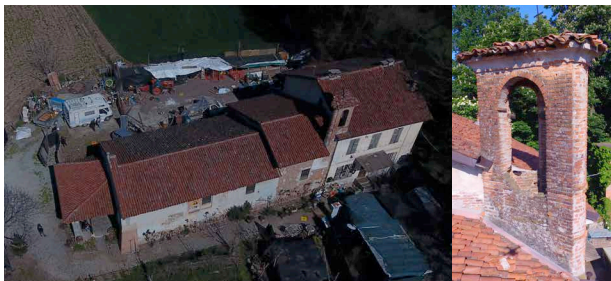
Figure 1 Aerial view of the church (left), belfry (right)
