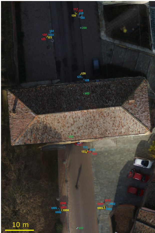
Figure 2. Points acquired. Station points (green), high-contrast signals (yellow), road cones (red), manholes covers (blue)
