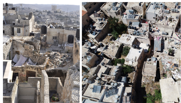
Figure 3: Landfills on roofs and courtyards.
