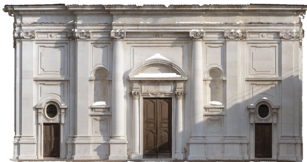
Figure 2. Ortho-rectified image of the Church.
