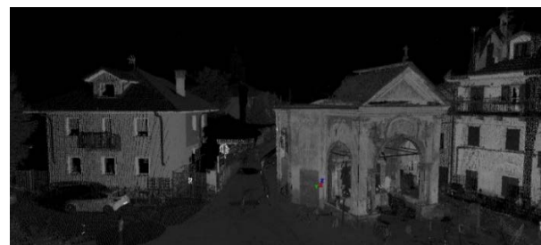
Figure 5: TLS (Leica C10 -10 scan stations) point cloud of Chapel two (architectural scale).
