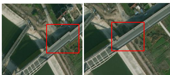
b. Bridge deformation
