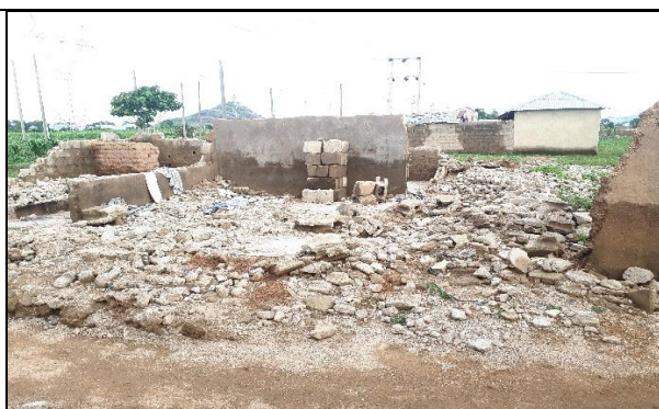
Figure 9. Completely Damaged building (Residential)
