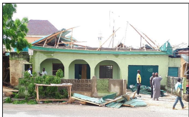
Figure 10. Completely damaged roof (Residential)
