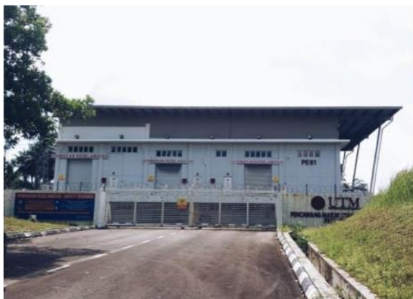
Figure 3: PE61 132/222KV Transmission Intake, UTM Johor Bahru, Malaysia
