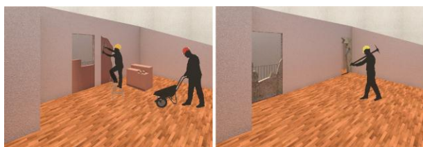
Figure 3. The variant represented the creation of two new doors and the closing of the existing ones by means of unstitch and sew.
