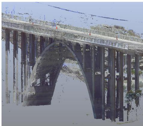
Figure 2: The texture-mapped point cloud of the Çayırhan Bridge. As already mentioned, a portion of the deck has been extracted in order to perform surface damage detection by using the
