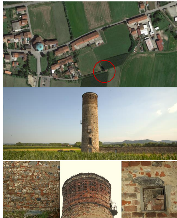
Figure 1. The late-medieval tower. Satellite image by Google©. Details on the dovecot and on mixed stone and brick masonry.
