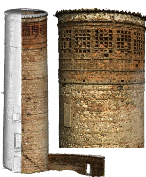
Figure 5. The 3D photogrammetric model and a zoomed image on the dense point cloud on the dovecot
