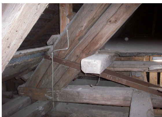
Figure 9. Photo of detail of the foot point of the Laves' balken .
