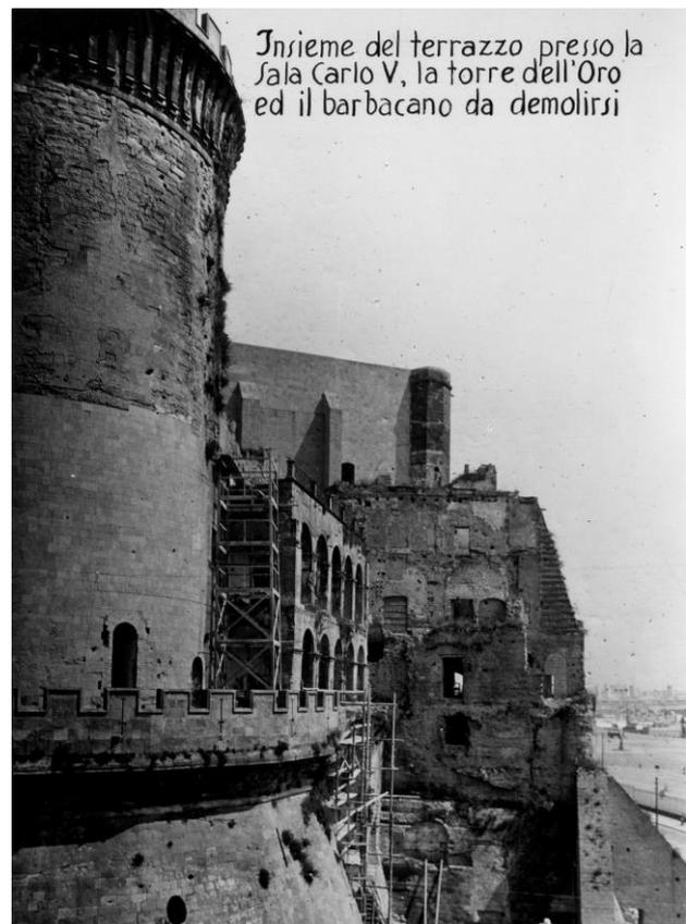
Figure 2. Castel Nuovo. The terrace at the hall Carlo V, the Torre dell'Oro and the *barbacane* to be demolished. In the foreground we can notice the repairs of the tuff truss performed for the lower part of the Torre dell'Oro (Archivio Storico Municipale Comune di Napoli, *Album 1, Patrimonio culturale, Castelnuovo prima e dopo i restauri*).
