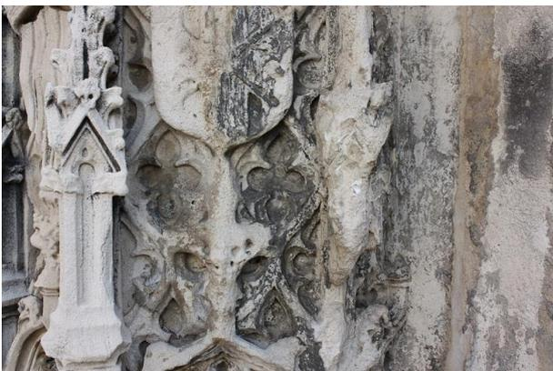
Figure 13. Castel Nuovo, Napoli. Internal court, near the entrance of Gran Sala, the detail of the degradation of marble decorations.
