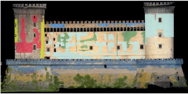
Figure 9. South Curtain: orthoprojection of point clouds processed by the laser scanner, colored with RGB data of photographs with detection for macro areas of degradation phenomena of Castel Nuovo, Napoli.
