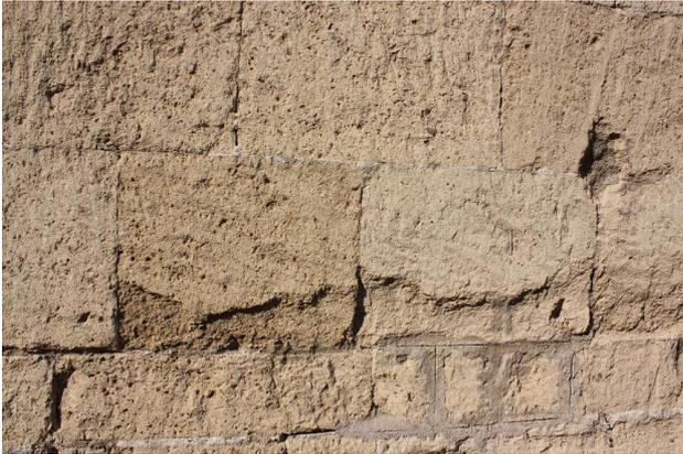
Figure 12. Castel Nuovo, Napoli. Internal court, southern perspective: phenomenon of alveolization and retraction for erosion of the tuff surface.
