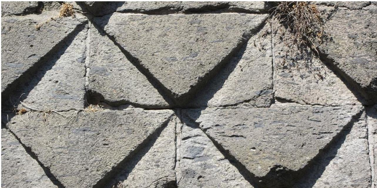
Figure 11. Castel Nuovo, Napoli. The coating in Piperno of *Torre della Guardia*. *The particular scale technique of the tower base.*
