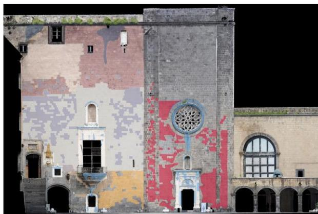
Figure 8. Inner courtyard, facade facing east: orthoprojection of point cloud elaborated by laser scanner, colored with RGB data of photographs with detection for macro areas of degradation phenomena of Castel Nuovo, Napoli.
