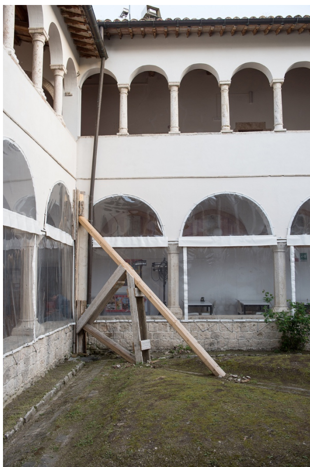
Figure 2. Emergency action for the safety of the main cloister after the earthquakes of August 2016
