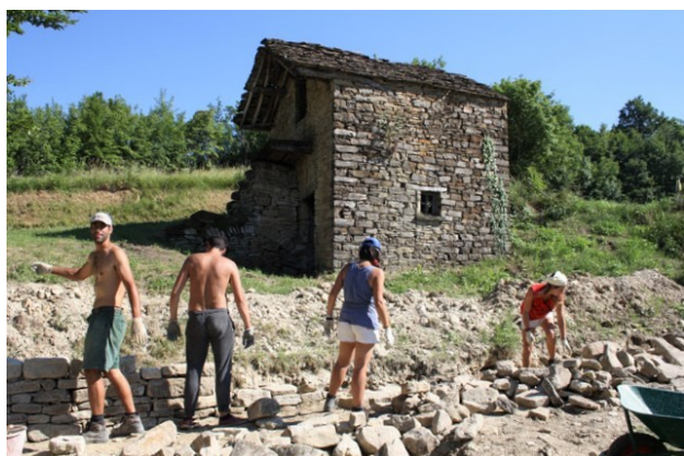
Figure 2. The construction of a dry-stone wall
