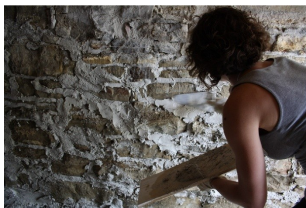
Figure 4. Use of natural hydraulic lime plasters
