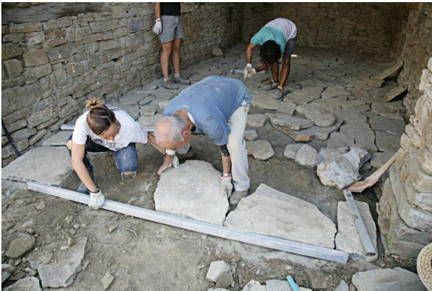
Figure 6. Laying a traditional stone floor
