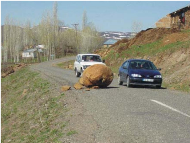
Figure 3. An example to rockfall from Bingol, Turkey, occurred after May 1 st , 2003 earthquake (MTA, 2003).
