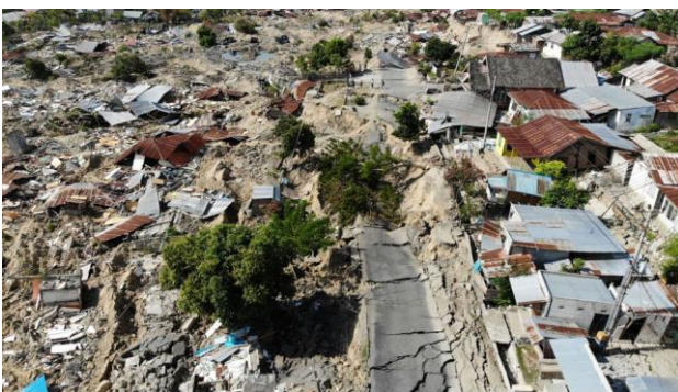
Figure 5. An example to liquefaction from Palu, Indonesia, occurred after September 28, 2018 earthquake, where shaking of the ground has caused roads to break up and houses to be swallowed (ref: news.sky.com).
