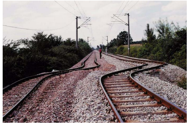
Figure 6. An example to surface rupture from Golcuk, Turkey, occurred after August 17, 1999 earthquake (Arpat, 2005).
