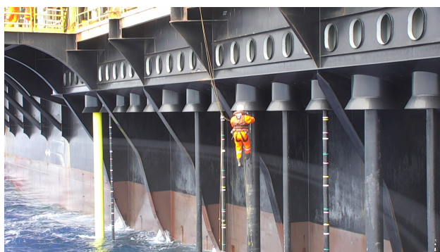
Figure 1. Industrial climbers inspecting the emerged riser section.
