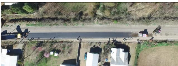
Figure 1. View on the construction site and machinery
