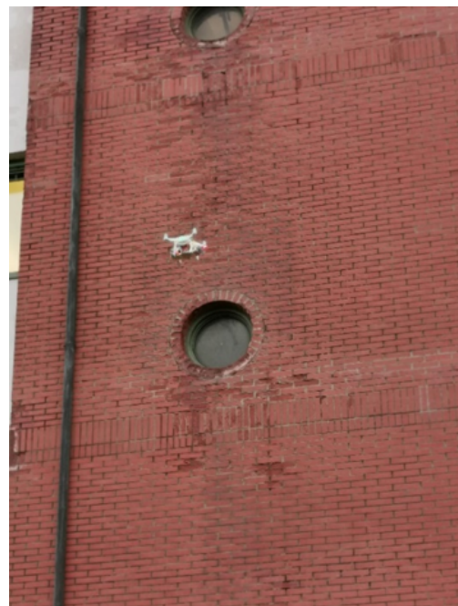
Figure 3. Drone flying close to the building façade.
