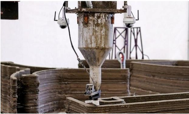
Figure 1. 3D concrete printer from PERI GmbH. Printable concrete is applied in layers and no formwork is required. Cameras are attached to the print head for visual monitoring of the printing process and results ©PERI GmbH (PERI GmbH, 2020a).
