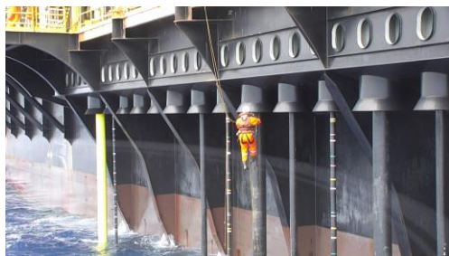
Figure 1. Riser inspection by industrial climber.
