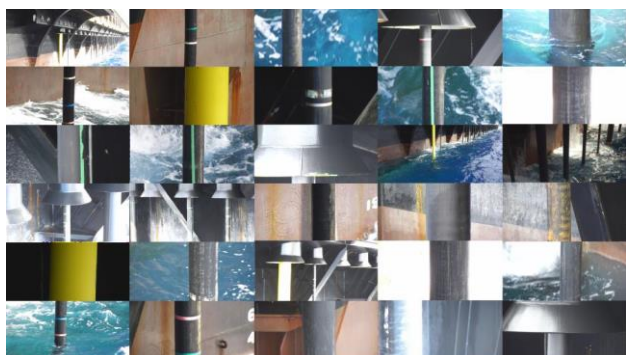
Figure 4. Real dataset for risers inspection process.
