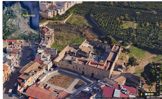
Figure 1. The Castle of Mareddolce (image from Google Maps©); unauthorized structures are still visible in this image.
