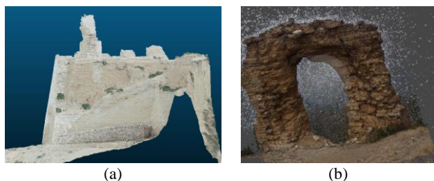
Figure 9. The generated DIM points of moon gate; (a) after collapse; (b) before collapse
