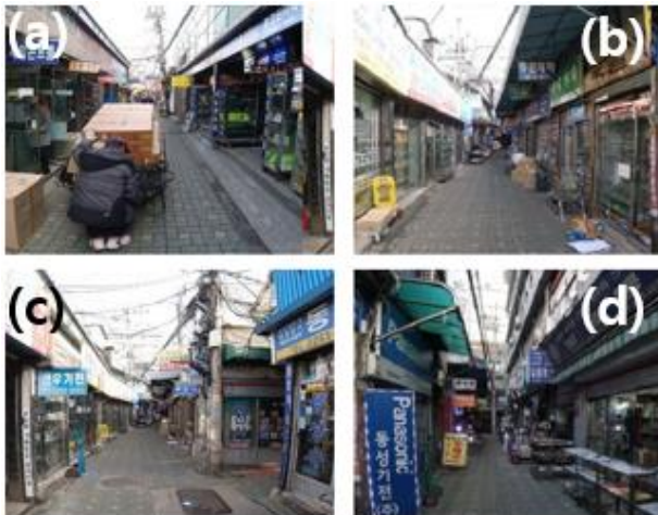
Figure 2. 4 pictures are the view of the alleyway. As you can see in pictures, the width of the road is very narrow. It is very easy to find telegraph poles, power lines and shading devices in the alley.
