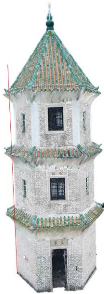
Figure 6. Diameter or the radius of the floor decreases at higher floor (the space between the red line and the prism at the floor increases for higher floor).
