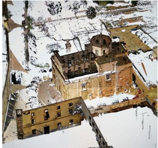
Figure 4. TLS reconstruction of the church and its neighborhoods.
