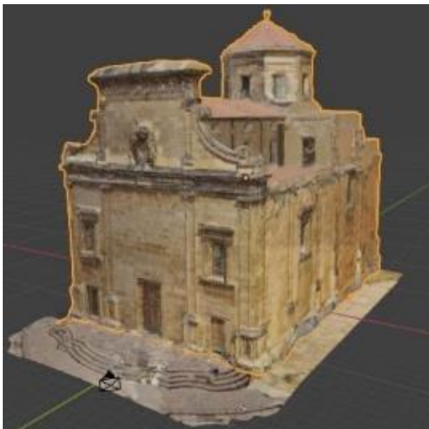
Figure 8. The textured mesh model of the church obtained following the second solution after editing operations in Blender.
