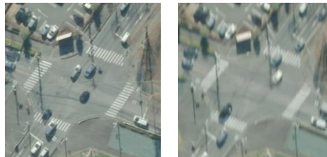
(c) intersection of roads
