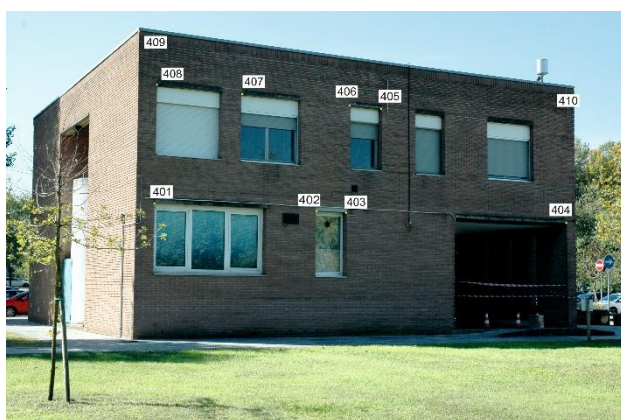
Figure 3. The ten points belonging to building's façade.
