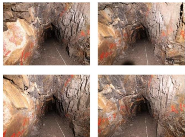
Figure 6. Example image of tunnel double-line parallel photography sequence.
