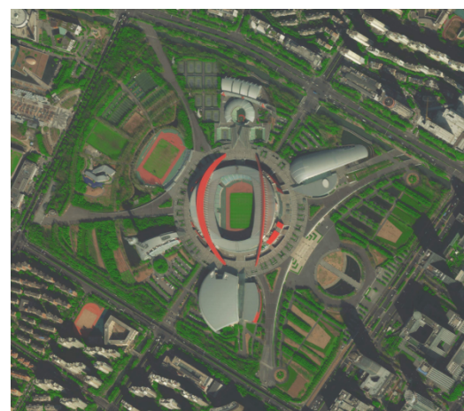
Figure 4. Top view of Nanjing Olympic Sports Center.
