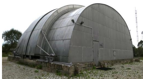
Figure 4. Building used for calibration tests.
