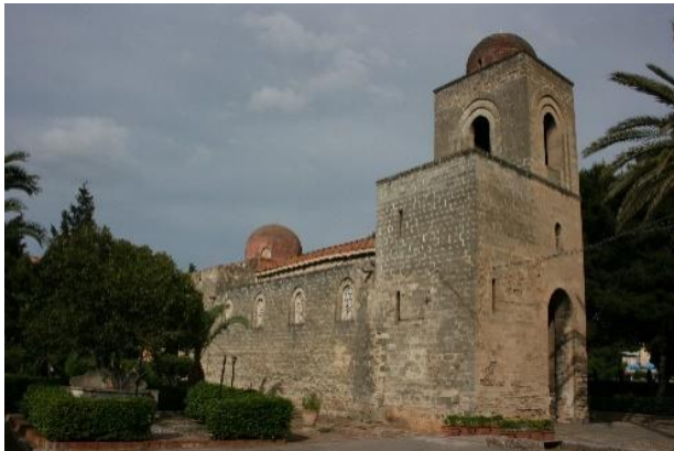
Figure 1. The exterior of the church.
