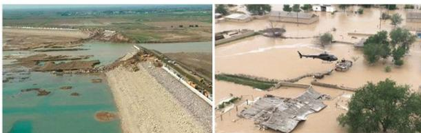
**Figure 2.** Views from the failure and the damages of caused by the Sardoba Dam break (photo credits: Fergana News, 2020)
