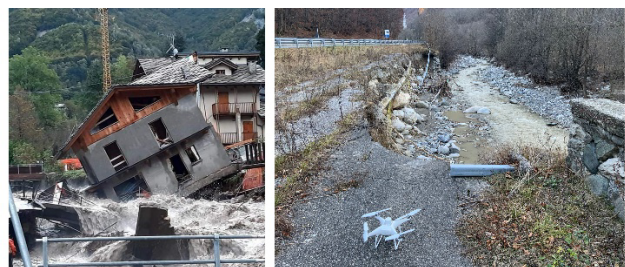
Figure 1. Some of the damages of October 2020 flood in the area of Limone Piemonte, Piemonte region, Italy.
