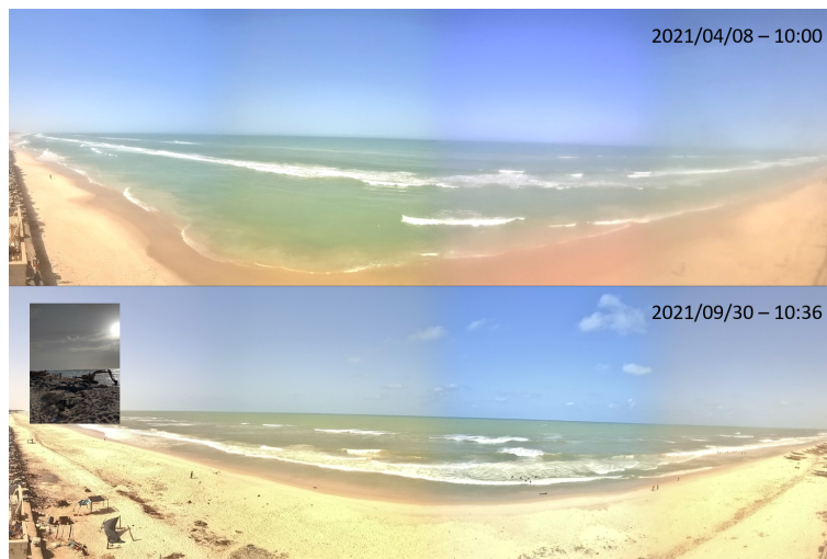
Figure 2. Images acquired with the camera (see Figure 1 for location) on the indicated time. A small picture (bottom panel, on the left) shows the on-going construction of the riprap.
