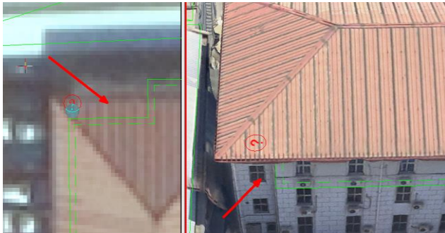
Figure 3. Position acquisition accuracy of permanent house exceeds the limit.
