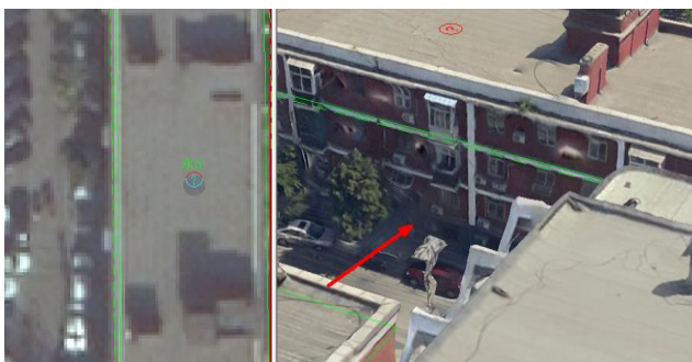
(a) The number of floors is wrong, and the fourth floor is wrongly filled as the fifth floor.
