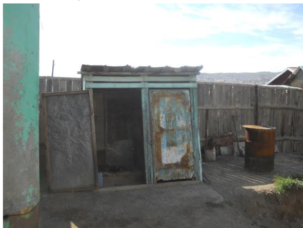
Figure 6. Pit latrines in ger area of Ulaanbaatar, Mongolia
