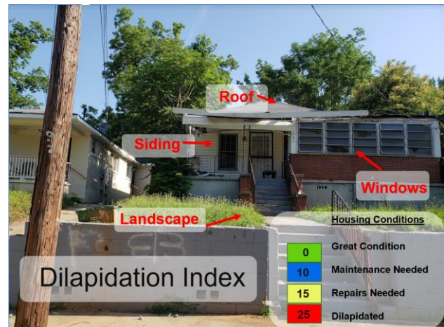
Figure 5. Example of a home along the BeltLine and the Dilapidation Index ranking system used when visually inspecting the condition of the front of the home.
